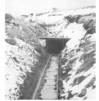
Ludworth Colliery adit on 1st March 1979, with a stream of orange water running out of the mine between the tracks.
