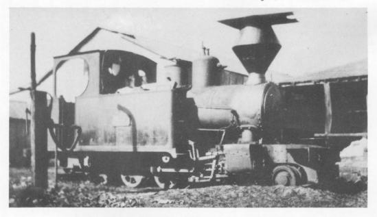
Cattle Creek Mill No. 2 LILY remained in virtually original condition apart from the 'balloon stack', here protected by a metal plate. However, it was later extensively rebuilt, including the fitting of an extended smokebox. (A. Carlson, G. Bond collection)
