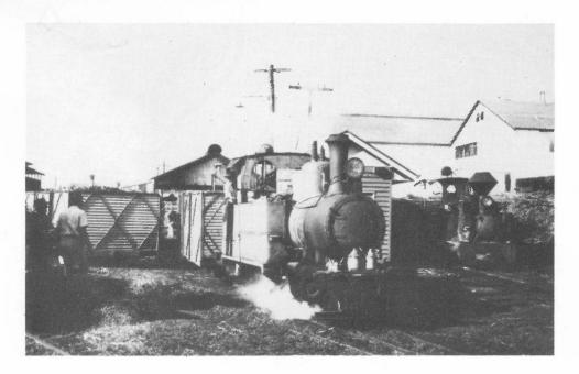
North Eton Sugar Mill No. 4 (HE 1239), shunts a rake of large bins used for machine cut cane. On the right is 0-6-0T No. 3, another Leeds-built engine from Hudswell Clarke, (HC 942/1911). (C.S. Small, G. Bond collection)
