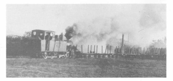
Invicta Sugar Mill INVICTA makes a smoky departure from the yard with a rake of cane trucks. This type, used for hand-cut whole-stick cane, has now been entirely superseded by bins. (P. Flecker, G. Bond collection)
