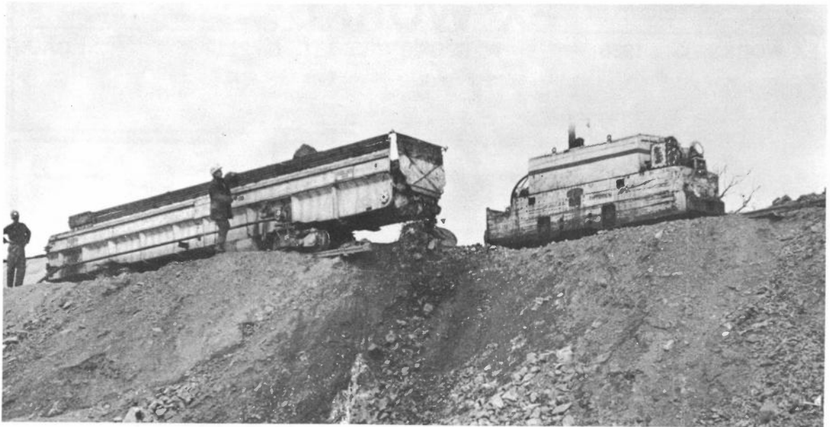
THYSSENS (GREAT BRITAIN) LTD, Tarn Moor Tunnel Contract, Helton Dale Site, Westmorland, 13/7/68 . . . . 2ft gauge 'Tunnel-car' built by AKTIEBOLAGET HAGGLUND & SONER of Sweden. This enormous bogie wagon empties its contents automatically by means of a built in conveyor belt. (air operated). In this picture, Greenwood & Batley 2862 (a 7 ton 4-wheeled Battery Electric) stands on a parallel track, having just hauled the loaded 'Tunnel-car' out of the nearby hillside (Pete Nicholson)
