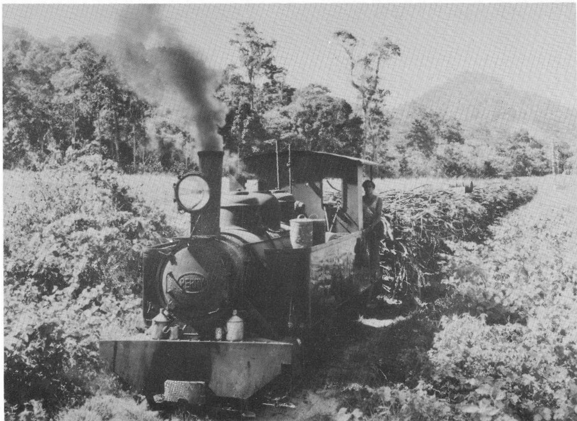
Tully Mill's No 7, a Perry 0-6-2T built in 1950 photographed hauling whole-stick cane during the 1950s. (The Courier-Mail, Brisbane)
