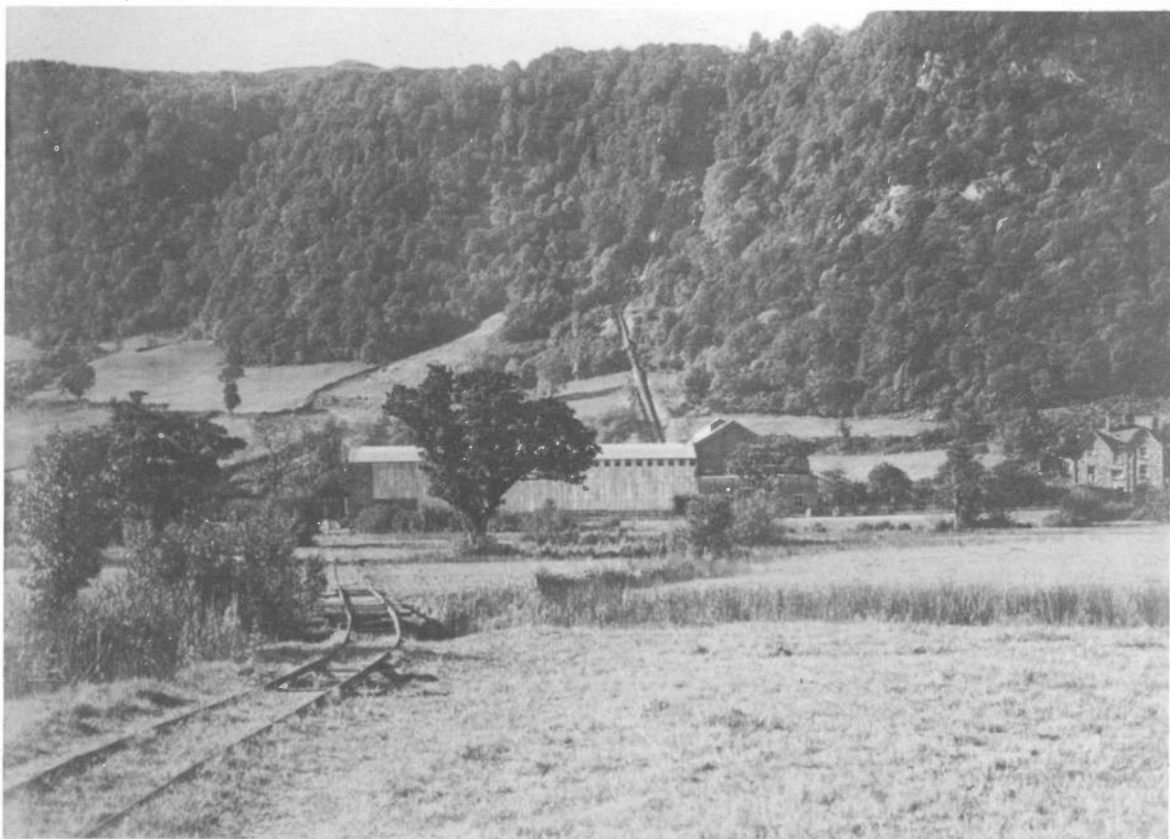
Dolgarrog works and the old power station about 1912. In the foreground is the line from the wharf to the smelter, and in the background the pipeline descends through the trees to the power station. (Central Electricity Generating Board)
