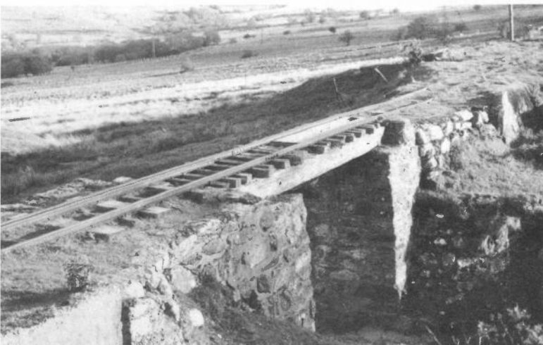
This simple bridge carries the rails over the path to the mine.
