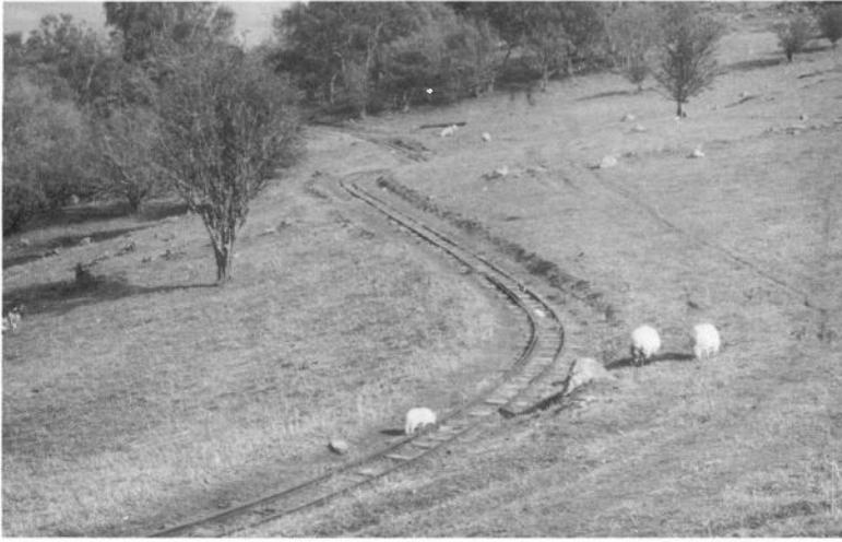
About ¼ mile beyond the incline head the track winds across this meadow, following the contours in true narrow gauge style.
