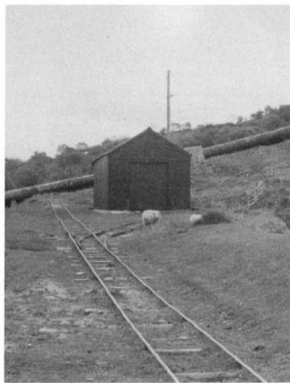
The locomotive shed near the incline head. May 1965. (P. Hindley)
