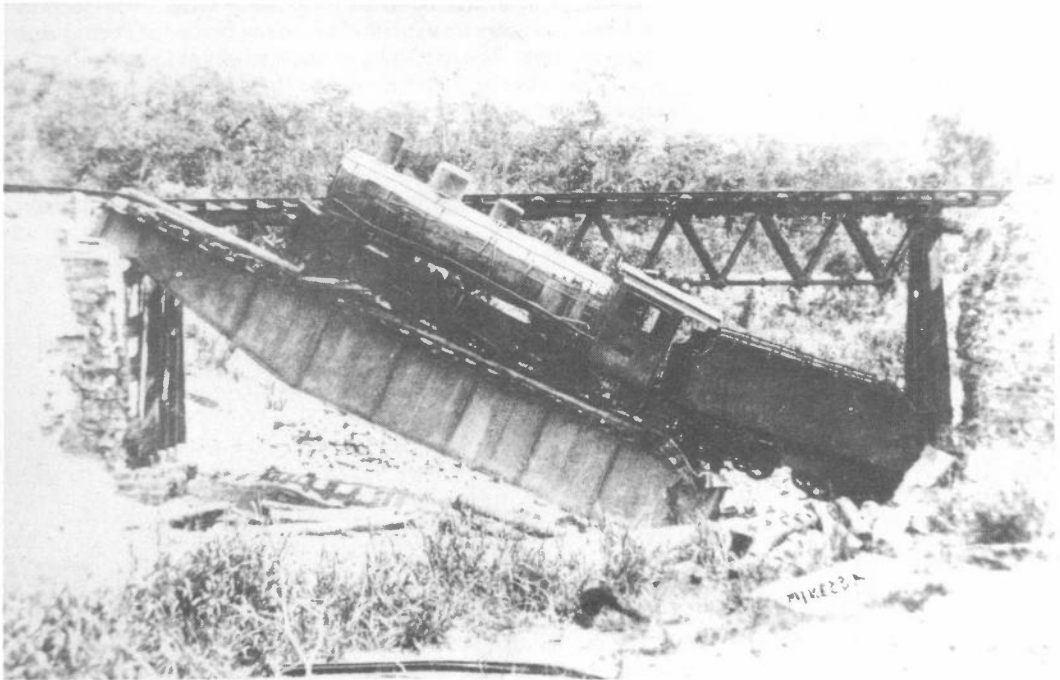
Hanomag 2-8-0 No 108 was run onto this demolished bridge at Mikesse. A diversion crosses the temporary bridge behind the loco.
