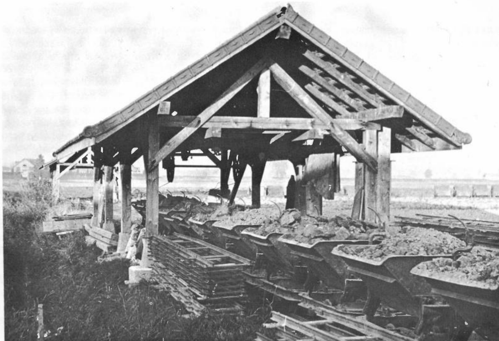
Tuilerie Corcelles. An ornate tiled awning covers the haulage terminal in the quarry. The curved rods guide the cable into the wagon fork. (R.A. Bowen, 10/1967)
