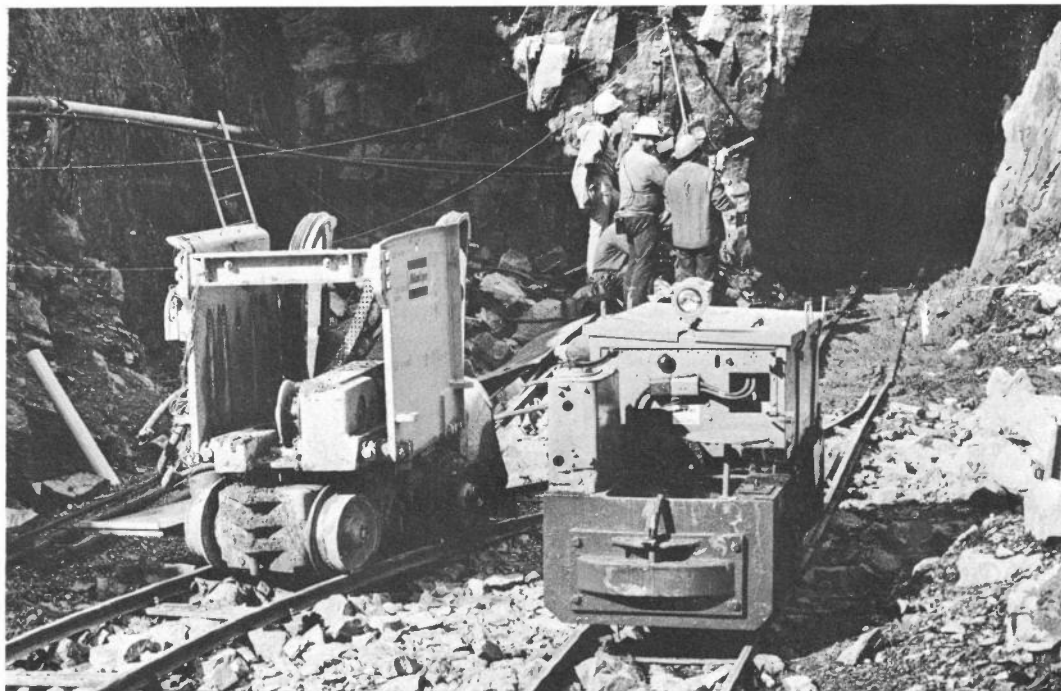
Latter days on the Festiniog Railway. The miners confer on the task ahead outside the new Moelwyn Tunnel in October 1975. In the foreground stand the Wingrove & Rogers battery locomotive and rock shovel. (P.J.G. Ransom)
