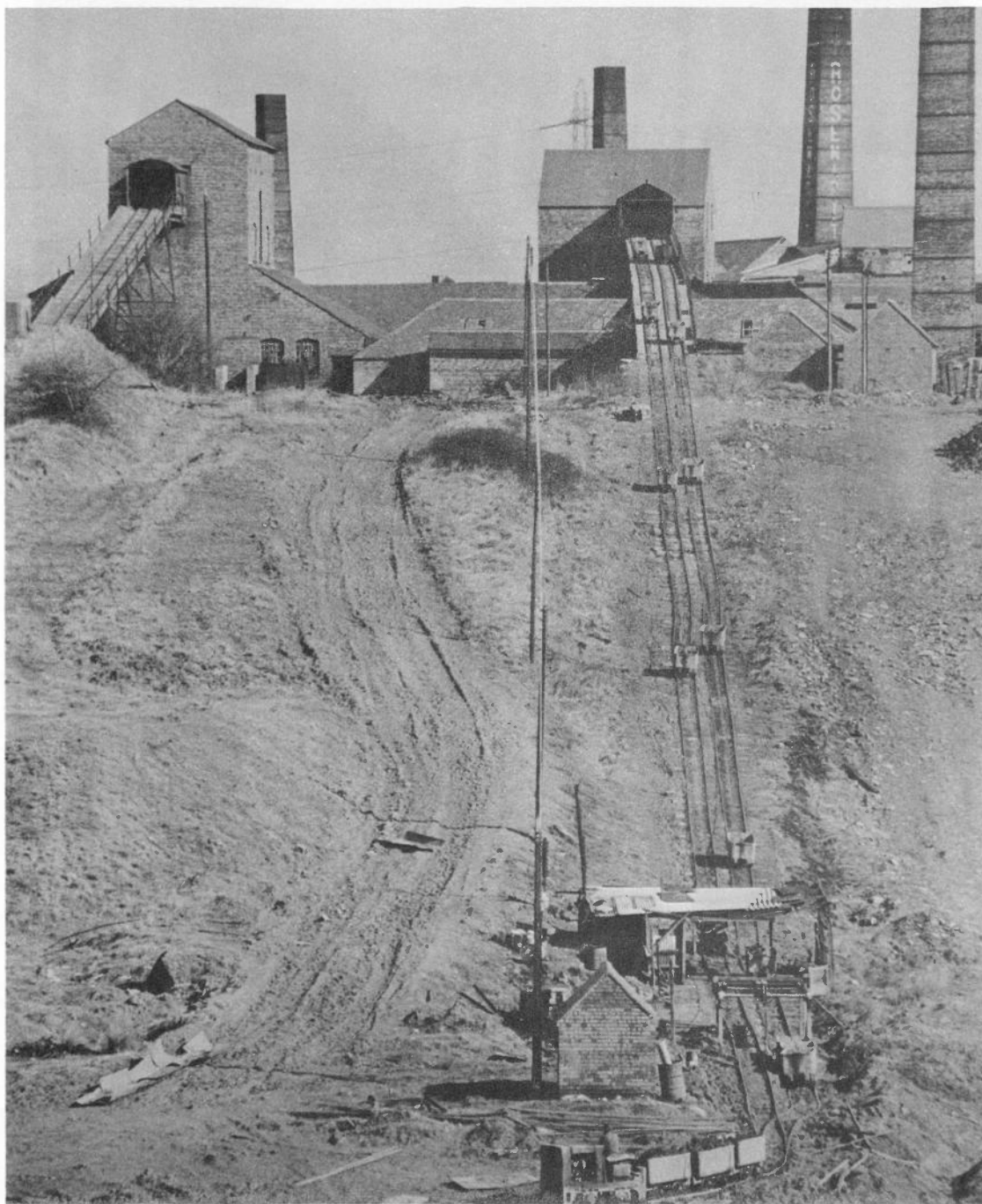
First Prize (Category E: Narrow Gauge 'Permanent Fixture') awarded to Peter Shoesmith of Birmingham. Photo: 2ft gauge rope-worked incline at the Rosemary Tileries of Haunchwood Lewis Brick & Tile Ltd., Cheslyn Hay, Staffordshire. 27th March 1970. Loco working bottom level is Ruston & Hornsby 4-wheel Diesel (L.B.U.) No. 432664 of 1959. Subsequently aquired for preservation by Pete Nicholson.
