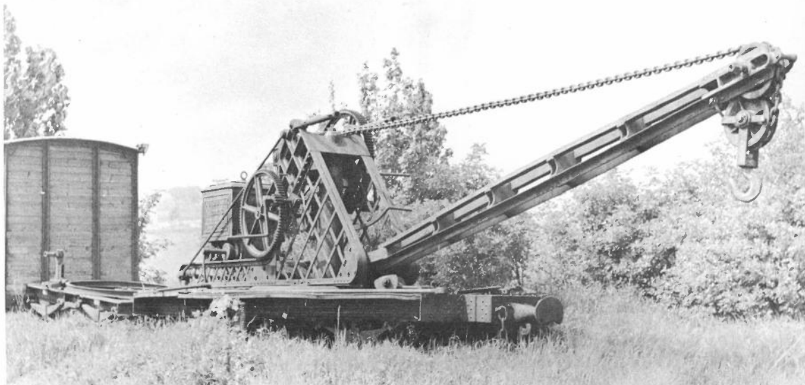
1st Prize — Category D (Narrow Gauge Rolling Stock). Awarded to Alan Bowler of Eastwood. Photo : C.F.T.A. Réseau de la Somme, France. Metre gauge vintage crane and match truck at St. Valery Canal in May 1966.
