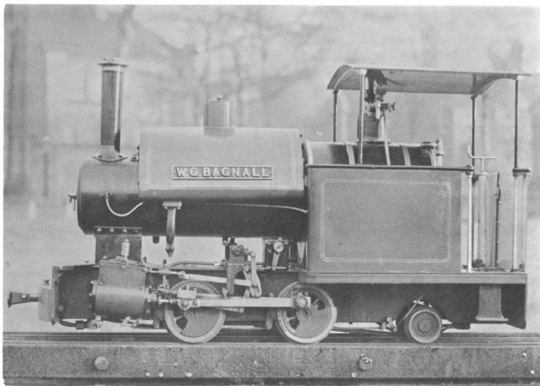
2½in gauge model of a 2ft 6in 0-4-2ST Bagnall. Construction of W. G. BAGNALL was commenced in the early 1920's and subsequently completed by Mr. S. A. Baker of Newcastle, Staffs in 1963. (Allan Baker)
