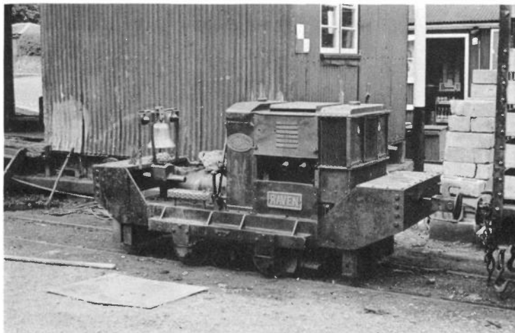
No.170374 (16/20HP) Probably the best known Ruston in the number range covered by this part of the Register, RAVEN at Llanfair Caereinion on the Welshpool & Llanfair. Since July '67 when this view was taken it has been 'retired' and its nameplates removed. The side extensions to the main-frame are distinctive of locos other than the basic 2ft gauge design. Note also the extended buffer beams (for W & L use) and that brass bell ! (Pete Nicholson)
