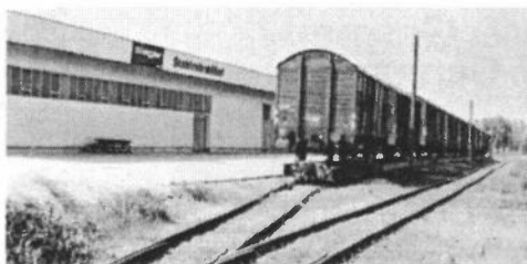
Transporter Bogiesladen with Standard Gauge wagonry, standing in factory siding near Schwarzach. (Helmut Mochel)
