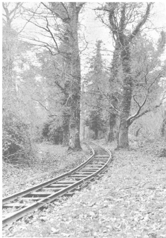
August 1969 : "Rough and ready" track as first laid. Platelayers from C.I.E. have since smoothed the curve and levelled out the humps. The tree on the left of the track was felled in July 1971. (A. G. Walsh)
