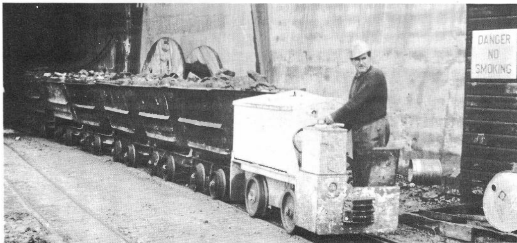
No.57 (Clayton 5590/F) – one of the Battery locos, emerging from the tunnel with six skips of spoil at 'Contract 120' on the bank of Loch Ness, 10/6/71. (Pete Nicholson)
